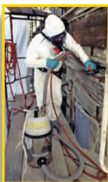
Attach power tools to a HEPA vacuum.
