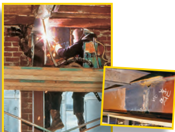
Strip back paint before cutting or welding.
